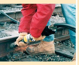
The GR60 Cup Stone Grinder was designed to meet rugged grinding needs while the HG60 Bull Nose Grinder is ideal for grinding and de-burring drilled holes in rail. The HG80 provides an ideal grinding tool from cleaning up a thermite weld to grinding a radius on frogs.
