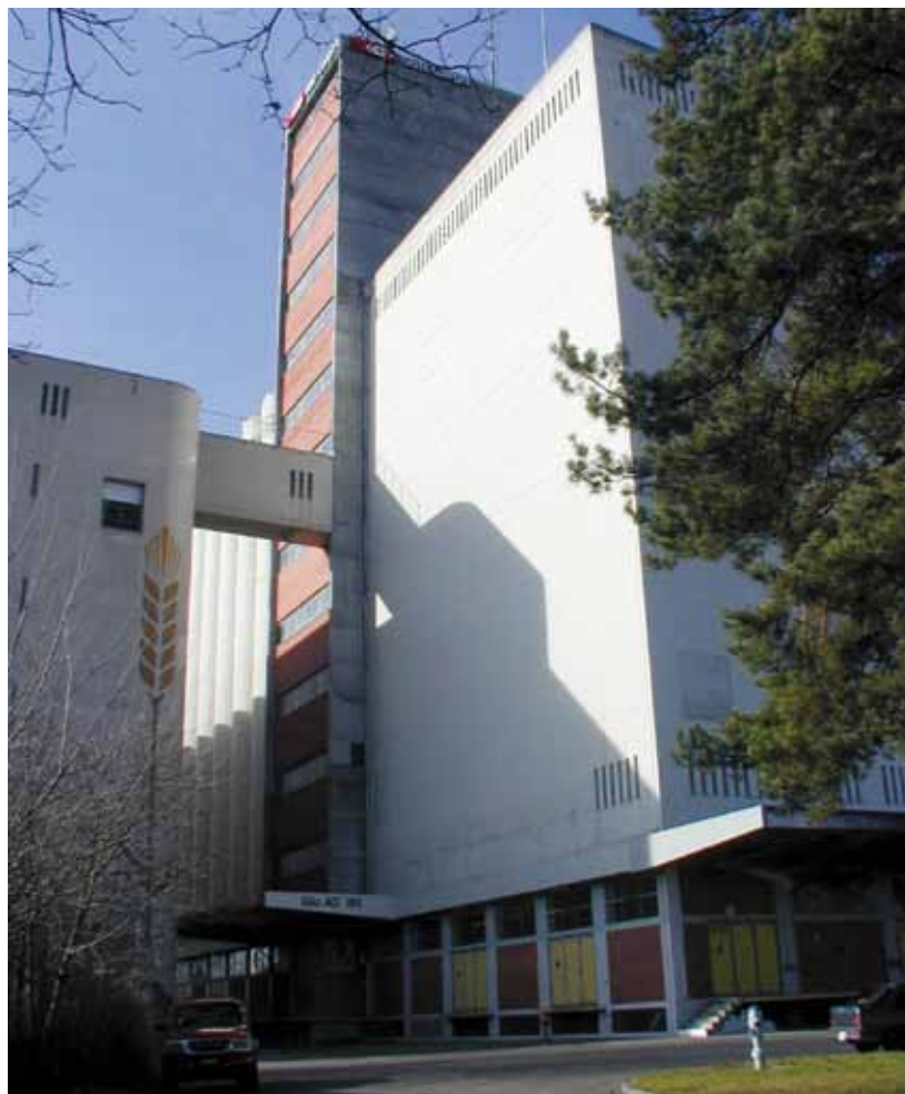
Silo AG Wil with a new technical inner life.
