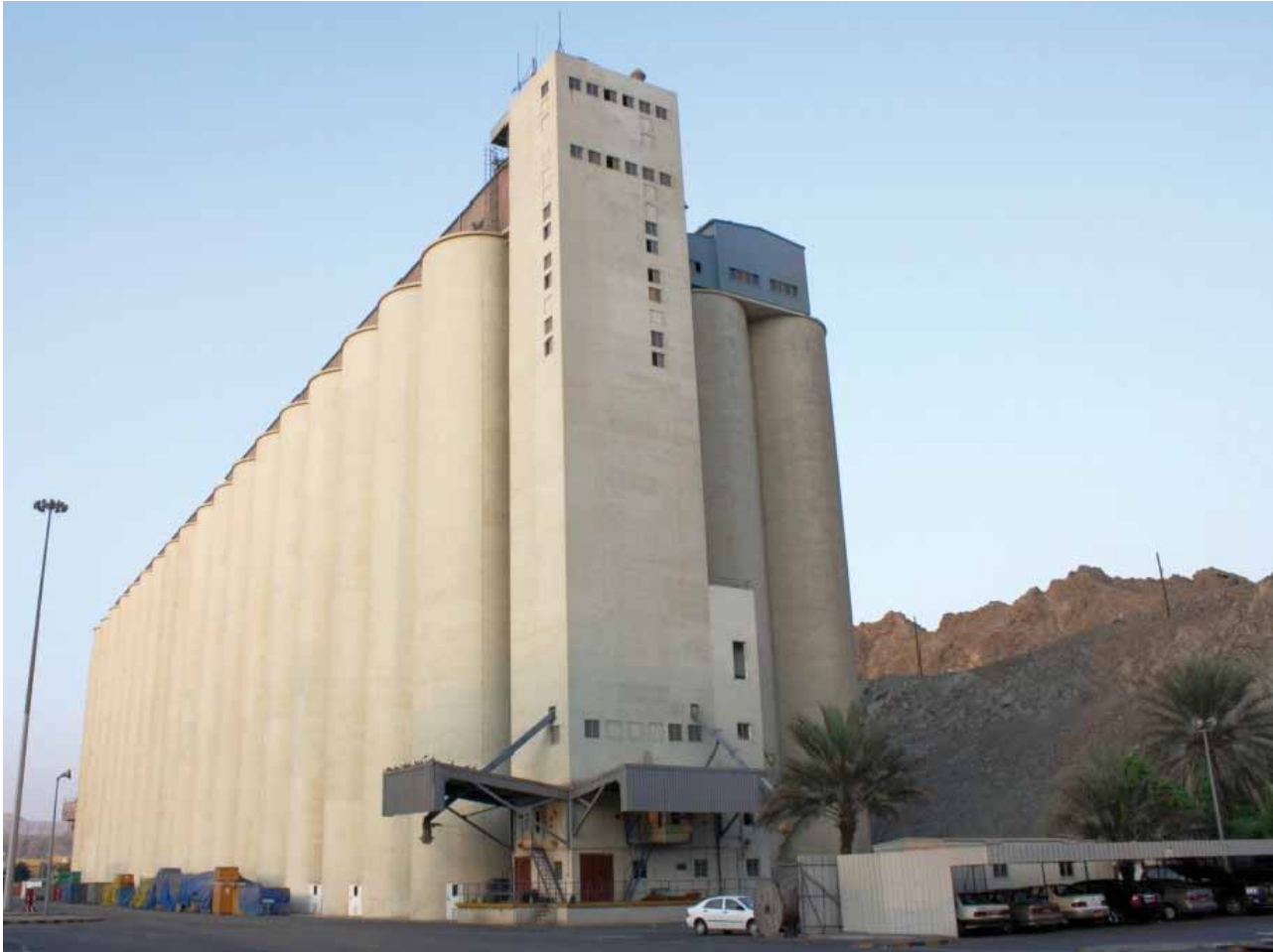
Oman Flour Mills Co.(S.A.O.G.), Ruwi/Port Qaboos, Oman, retrofit of existing silo facility.
